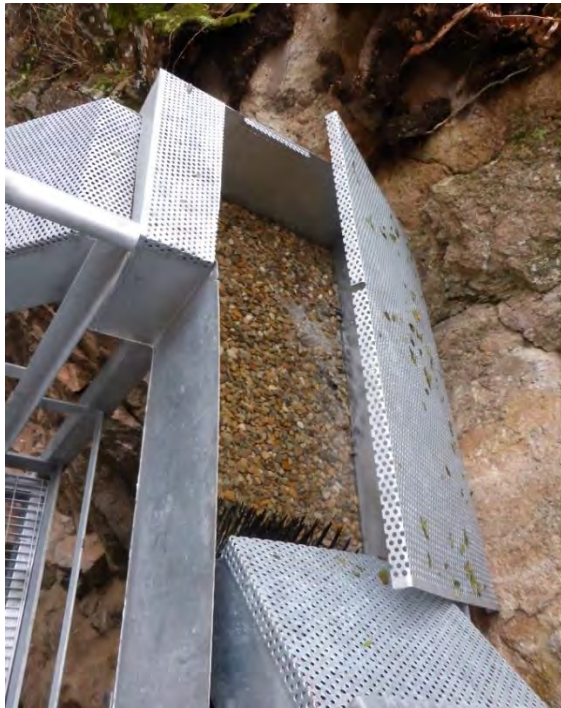
REST POOL FILLED WITH GRAVEL (LEFT) AND CHANNEL NEXT TO MONITORING CABIN
